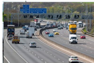
Motorway mode/ Smart motorway
