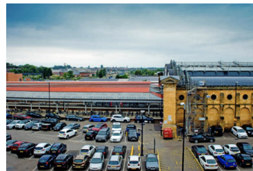
Railway station/ Transport hub
